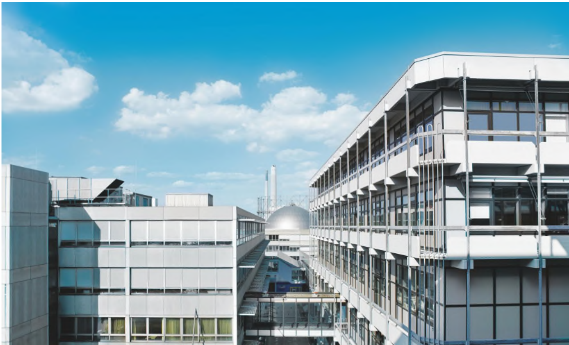
The headquarters of Witzenmann GmbH in Pforzheim (image source: Witzenmann)
