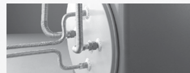
Fig. 3.4.9 Sample installation of device pipework with flexible annularly corrugated hoses
